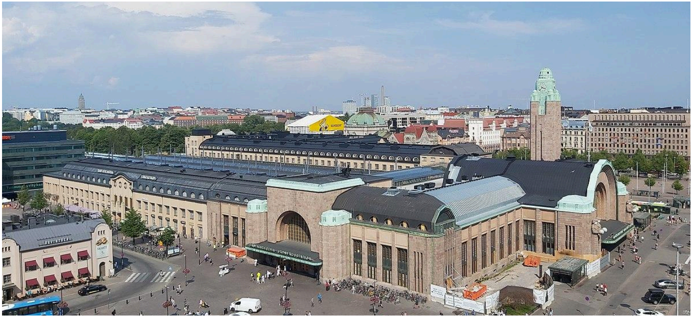
Central Railway Station of Helsinki
